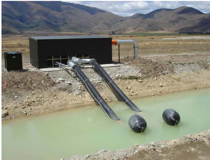
Typical structure used to pump water from an irrigation race to a farm
